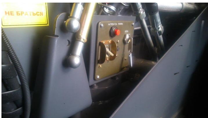
Pre-start heater control panel is located under the hood, to the left in the direction of tractor travel, behind the cooling unit.
